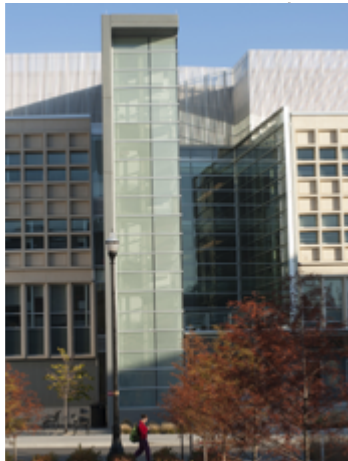
Cunz Hall renovation
